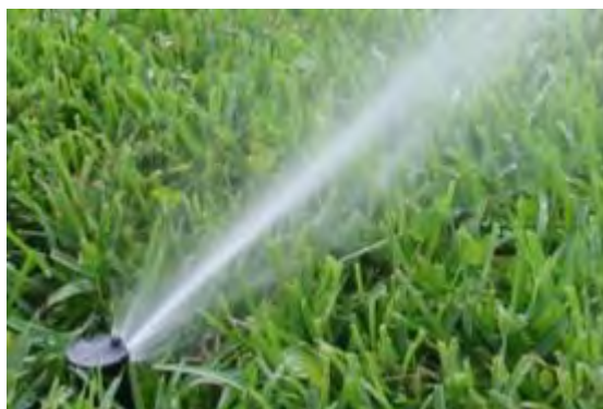
Figure 41. Rotor used to irrigate open areas of turf.
